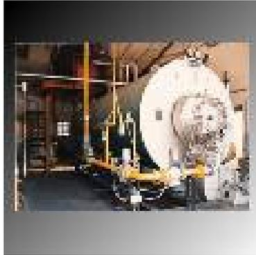
the steam and heat exchange surface. To put it in context. A water film on the wall of the heat exchange surface is 60–70 times more resistant to heat transfer than the iron or steel wall of the heating surface. (and 500–600 times more resistant than copper!!)
