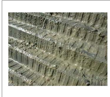
A calcium carbonate / biofilm deposit on the inside of a cooling tower pack
